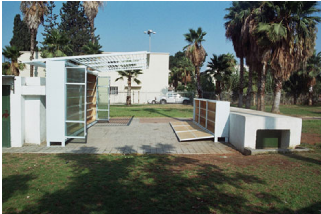
Figura 7. Levinski Garden Library. Autor: Yoav Meiri Architects. Fuente: Yoav Meiri Architects
