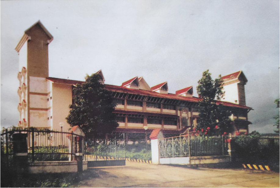
A future proof facility with plug and play type of LAN, into which about 300 systems can be plugged in, with digital storage systems, Internet Servers, ICT training facilities etc built by Dr. Michael in 1997 to house KAULIS headquarters and other ICT Systems.
