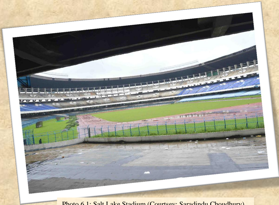
Photo 6.1: Salt Lake Stadium (Courtesy: Saradindu Choudhury)
