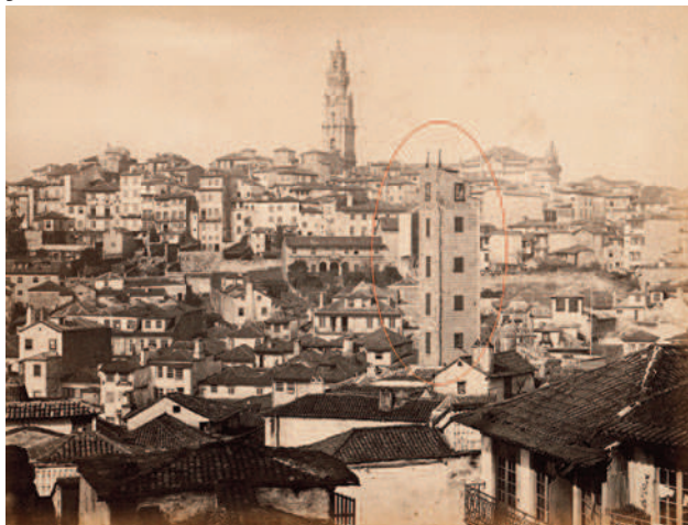
Figure 9. Photograph 2618 (Oporto, view from the Cathedral). Circled in red is the tower of the lead factory, which disappeared at the end of the 1860s. (José Manuel Martins Ferreira Collection).
