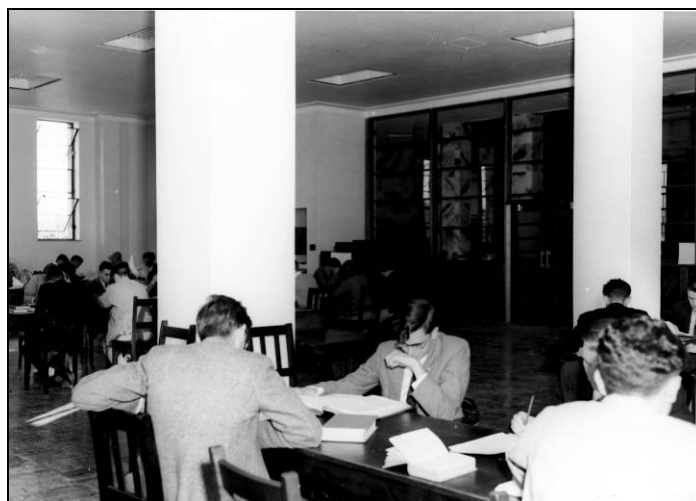
Reading Room (Ground Floor)
