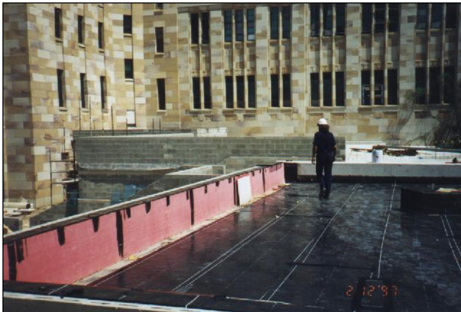
"The Link" under construction, December 1997
