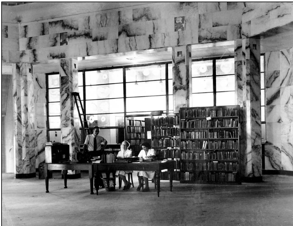
Settling in at St Lucia, about 1949 Ground floor of the Main Library building at St Lucia (now Level 2 of the Duhig Building), probably just after the move from George Street. The man standing is apparently Harrison Bryan. The older woman is probably Nellie McIver.
